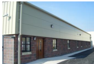
An Post, Delivery Service Unit
